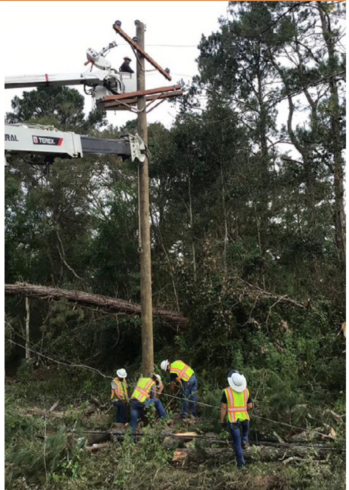
NOEC lineworkers replace a damaged pole
